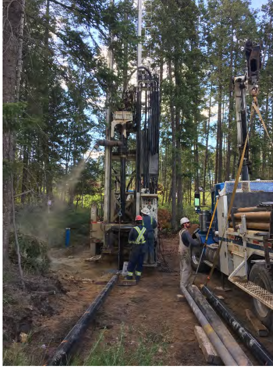
Photograph 3. Drilling of MW18-11 located on the SW corner of the Golden Landfill outside of the landfill perimeter (June 2018)
