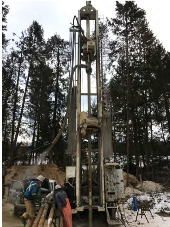
Photograph 5. Drilling of MW18-11 located on the SW corner of the Golden Landfill outside of the landfill perimeter (December 2018)
