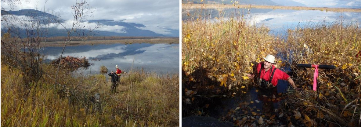
Figure 17. Photos (left to right): DLNA south cross dike inspection October 30, 2016, showing large beaver lodge (potential cause of wetland water retention issues, if beavers have burrowed through dike and impacted structural integrity of dike); Marc-Andre Beaucher standing in beaver tunnel (~50 cm deep) which appears to go into the dyke.
