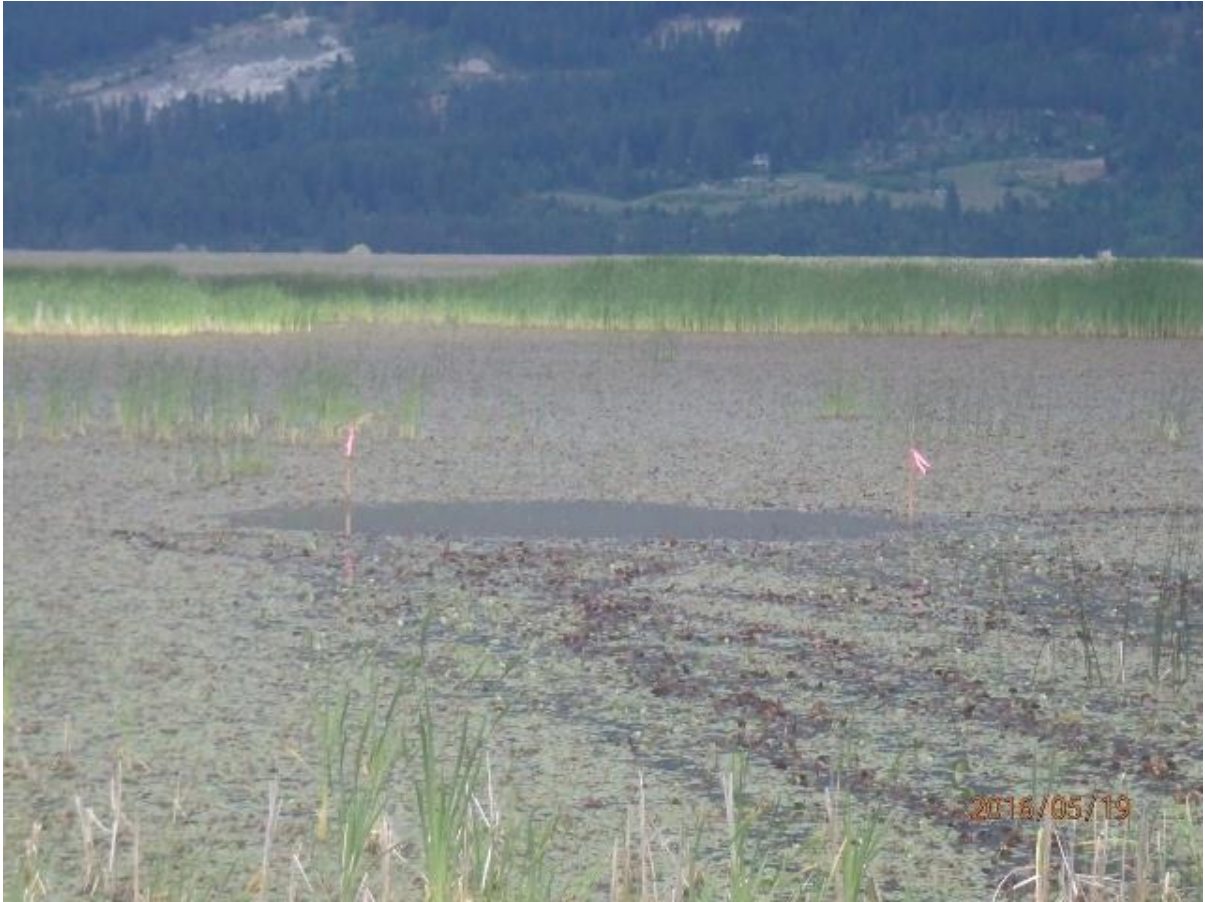
Figure 18. Photo of watershield removal test plot upon completion May 19, 2016.
