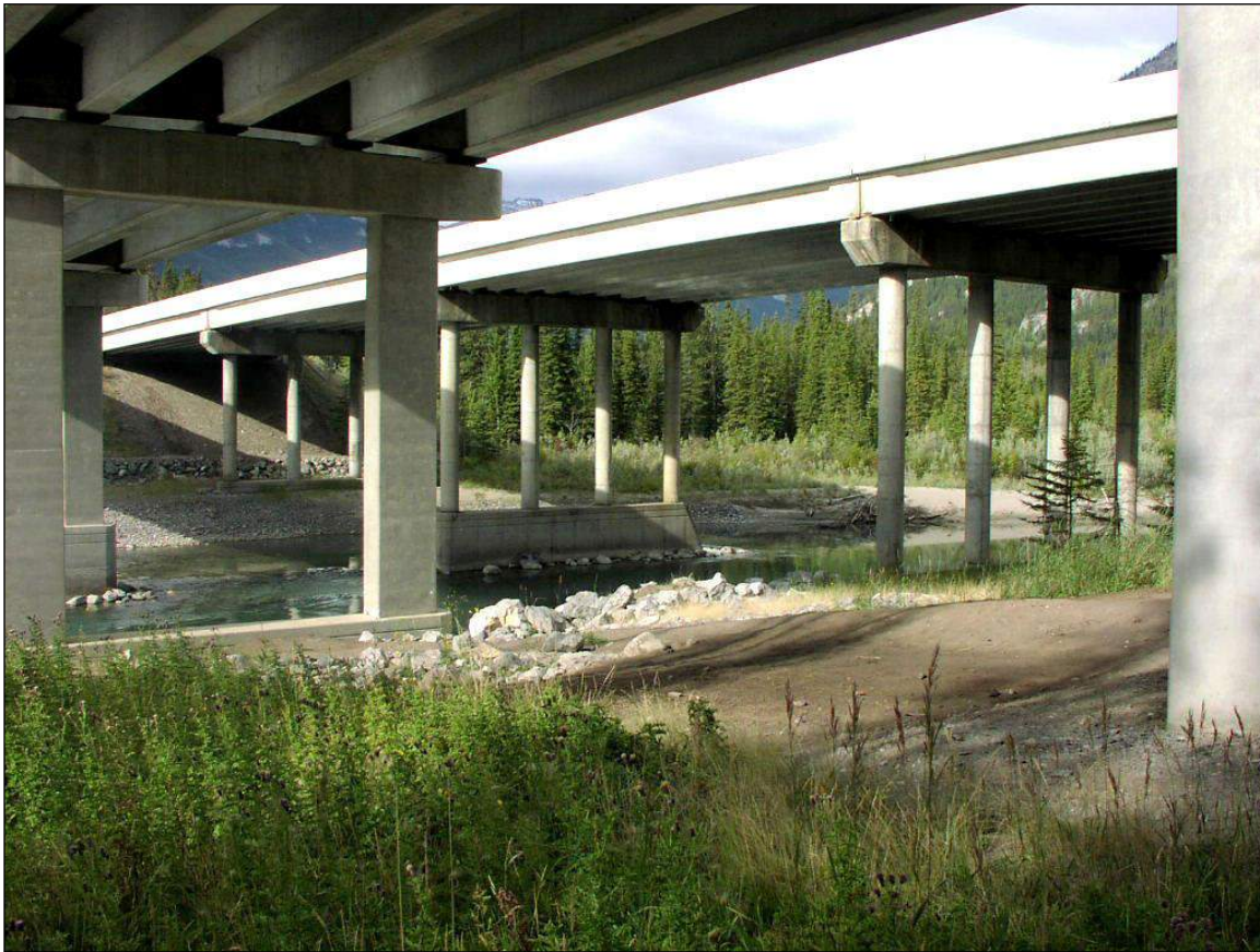
Large span bridge with retention of riparian vegetation (Credit: Tony Clevenger).
