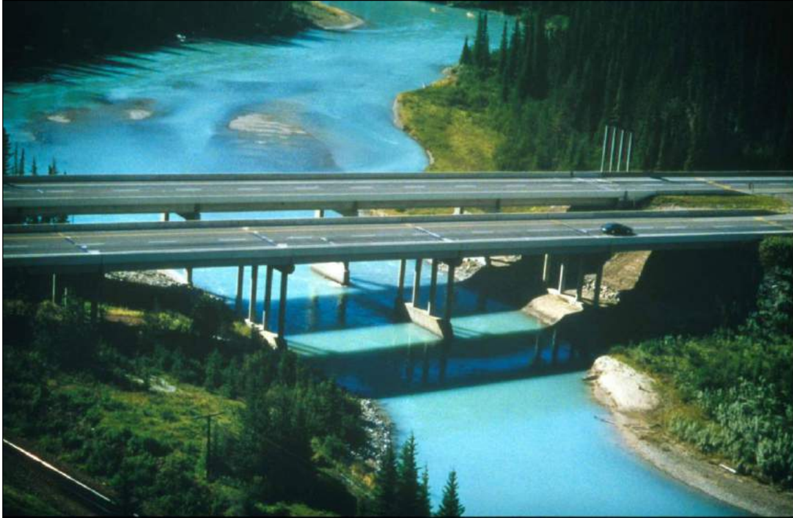
Large span bridge designed to conserve floodplain (Credit: Tony Clevenger).
