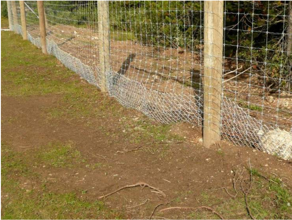
Wildlife exclusion fence with buried apron (Photo: Tony Clevenger).
