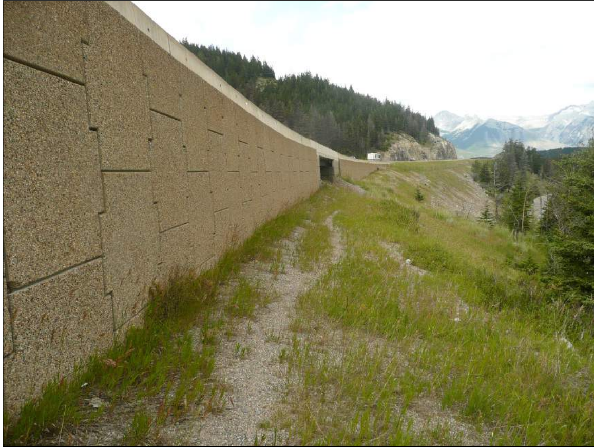
Mechanically stabilized earth (MSE) wall serving as wildlife exclusion “fence” (Photo: Tony Clevenger).
