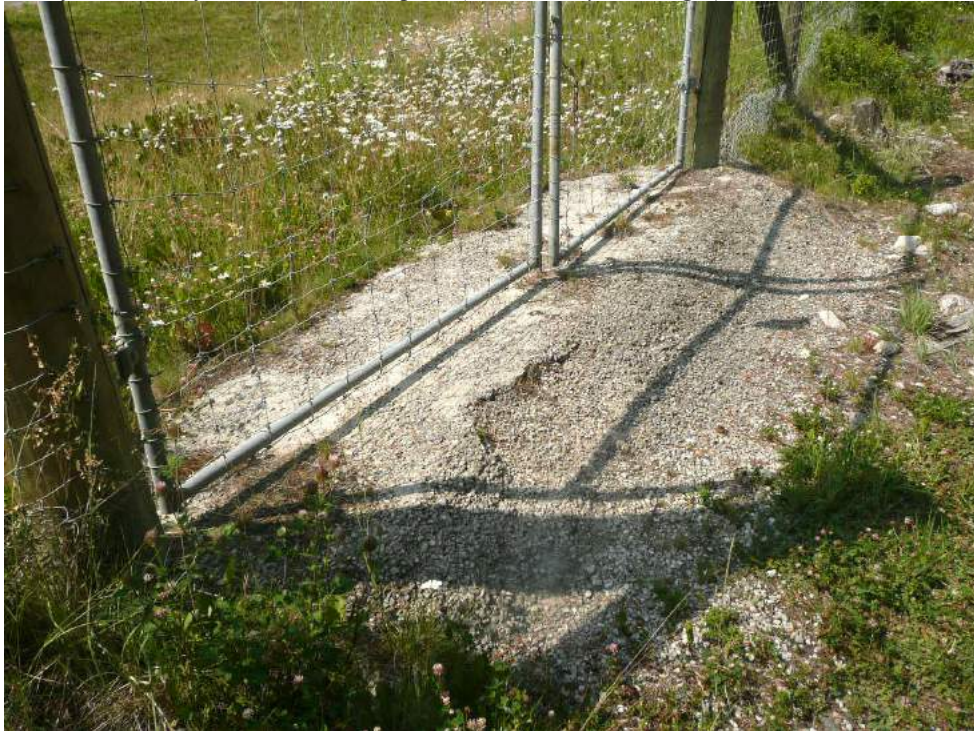
Concrete base of swing gate to prevent animal digging under wildlife fence (Photo: Tony Clevenger).
