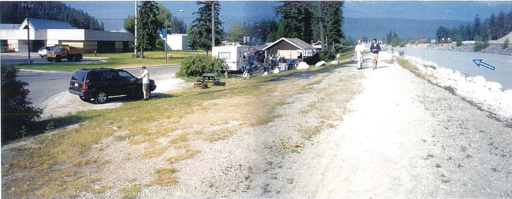
1. Entrance to campground looking downstream. The dyke crest is 4 m wide at the top with a 1.6 m drop to the ground level beside the road. Potential breach area to evaluate.
