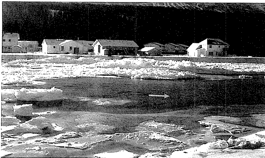
A11. 1995, looking at River Glen (Section K6 to K6a) from north bank. Ice shove approaching top of dike level in places.
