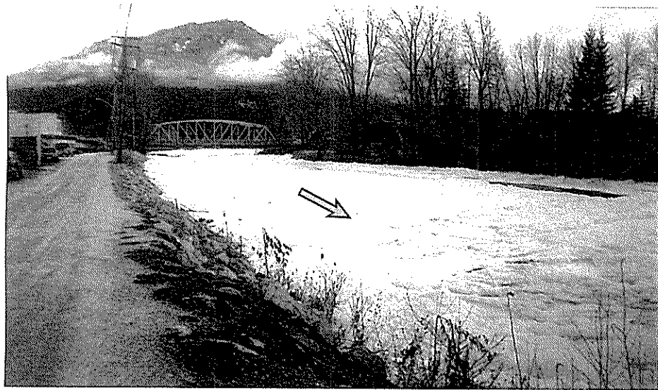
A13. December 1997. Looking upstream towards Highway 95 bridge. Ice shove within 2m of top of dike. Water level more than 1 m lower. River discharge only 8 to 13 m 3 /s at the time.
