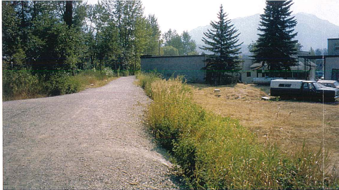
5. Looking upstream along dyke beside sub-channel downstream of Highway 95 bridge. Significant drop to natural ground of approximately 1.5 m.
