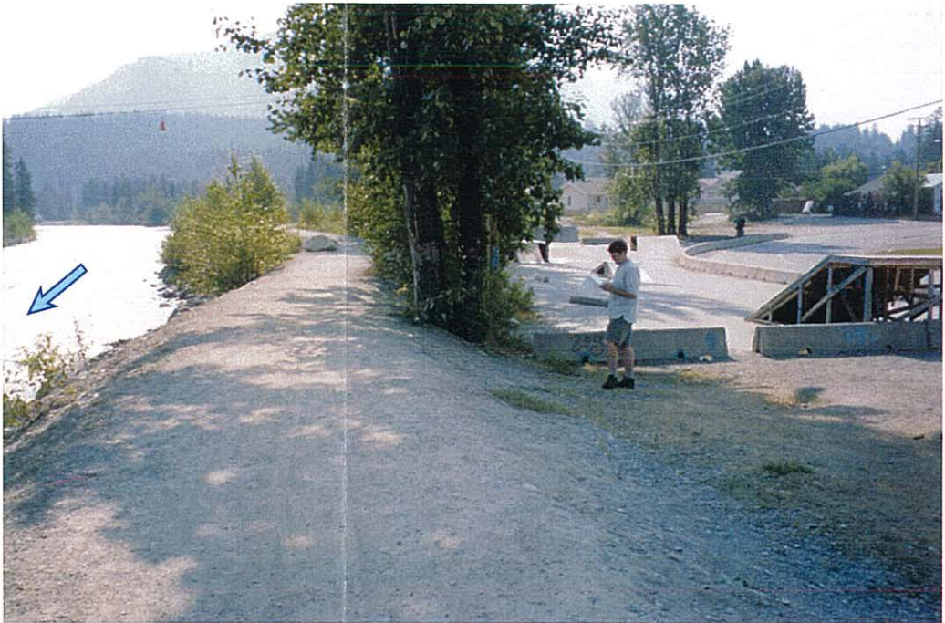
4. Skateboard Park looking upstream. The dyke crest is 0.96 m above the ground in the park area and 1.4 m above the road with a crest width of 3 m. The river side of the dyke is slightly steep at 55%. Potential breach area to evaluate.
