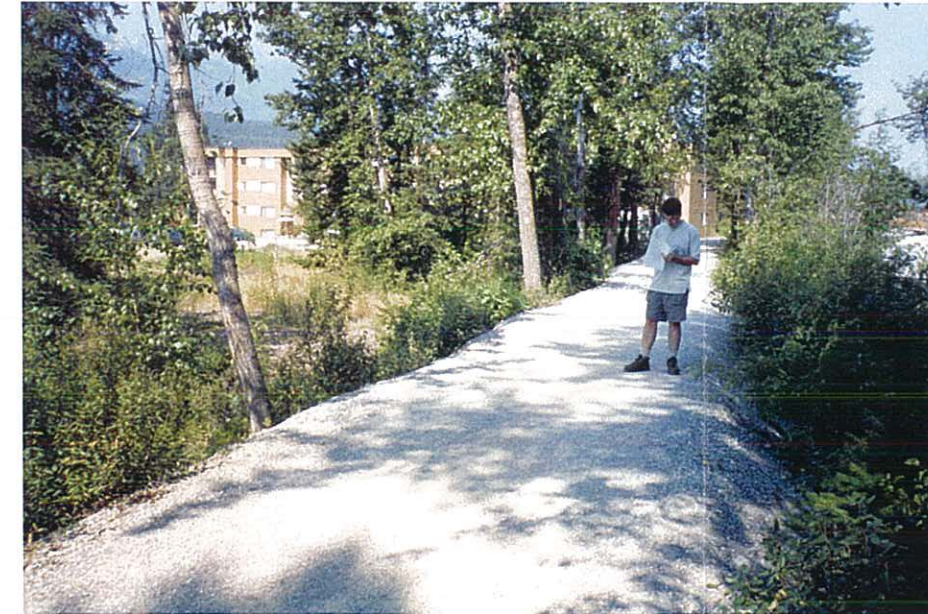
6. Looking downstream from location of Photo 5. The narrow 3 m wide dyke crest is 1.8 m above the natural ground level. The landward slope of the dyke is oversteep at 62%. Dyke upgrading is planned along this sub-channel reach in September - October, 2003.
