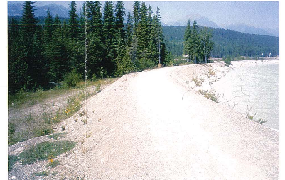
9. Photo taken halfway between Section K7a and K7b looking downstream. The 5 m wide dyke crest is approximately 3 m above natural ground level.
