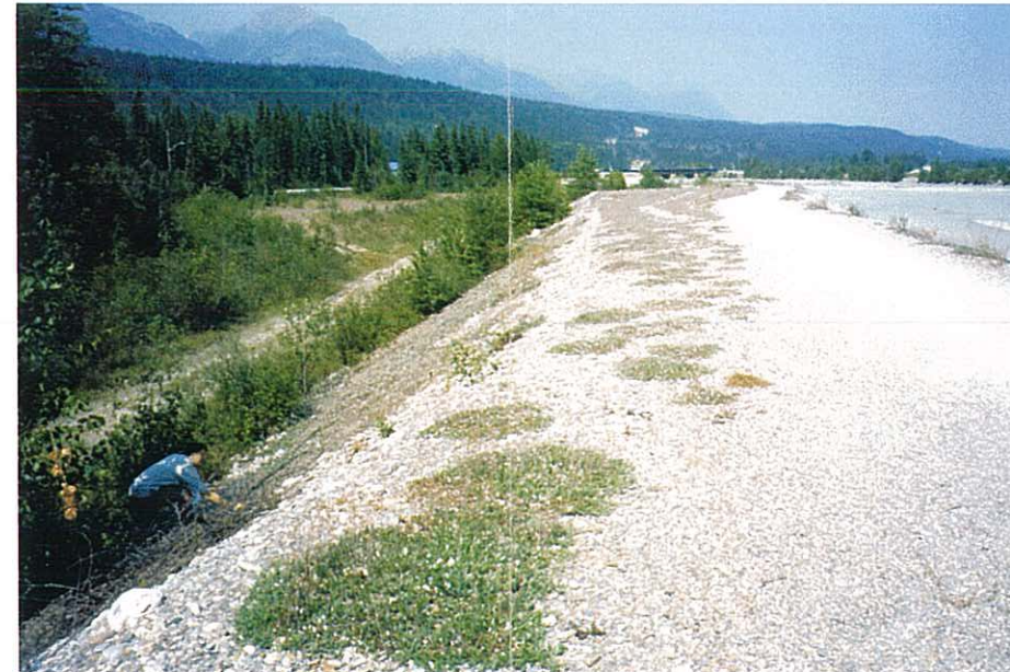
8. Photo taken from near Section K7 looking downstream. The 6 m wide dyke crest is 3.4 m above the natural ground on the left.
