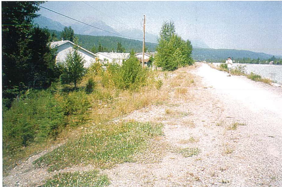
7. Photo taken from near Section K6 looking downstream. The 6 m wide dyke crest is 1.7 m above the natural ground on the left. The natural ground on the left is a local depression. Residential area ground level is about 1 m below the dyke crest.
