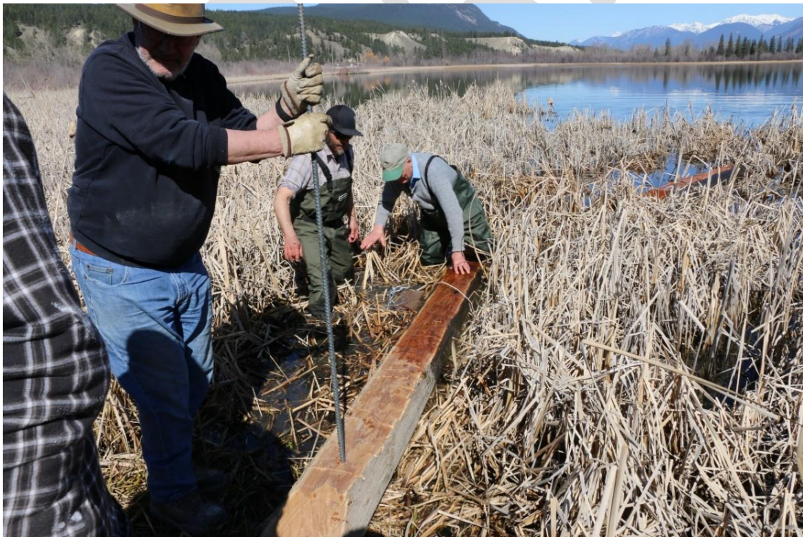
Figure 3. Securing a basking log near the shoreline using rebar pounded through the log and into the ground.
