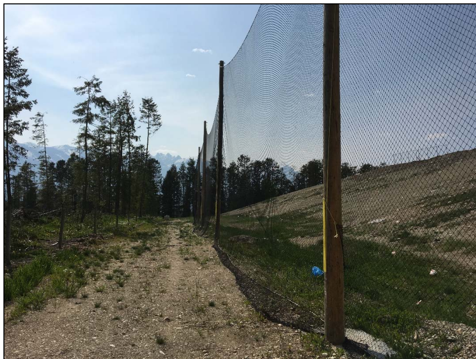
Photo 6: Litter Control Netting Along Southern Property Boundary
