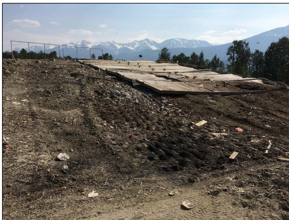
Photo 7: Steel Plates Used for Daily Cover and Portable Litter Control Fencing the Background
