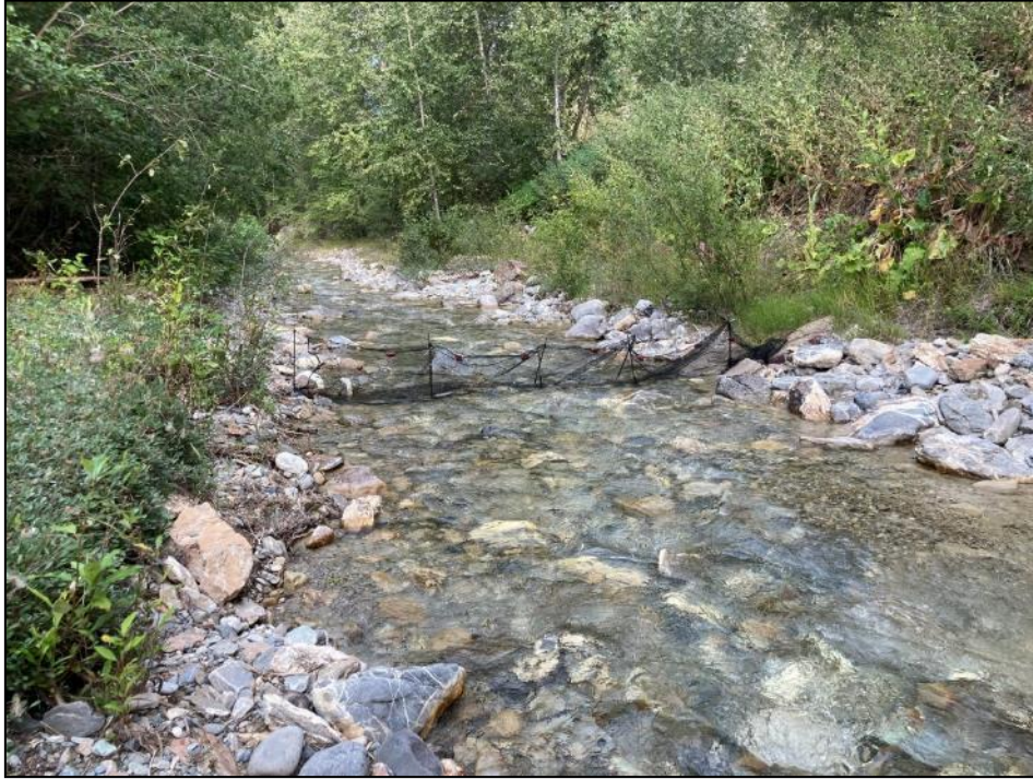
Photograph 3. View downstream, upstream exclusion stop net at Hospital Creek prior to instream works. August 21, 2022. Hospital Creek Bank Restoration and Protection – Fish Salvage.
