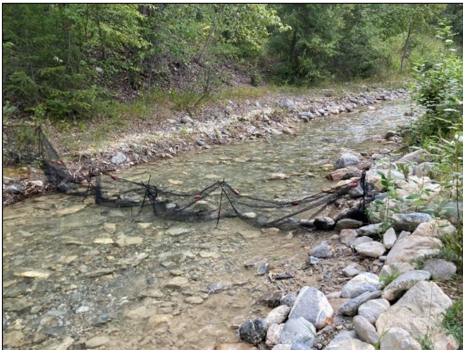
Photograph 4. View upstream, downstream exclusion stop net at Hospital Creek prior to instream works August 21, 2022. Hospital Creek Bank Restoration and Protection – Fish Salvage.
