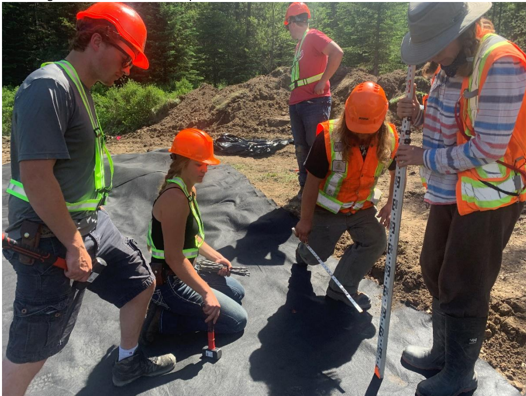
Figure 17: Crew helping lay a fish-grade pond liner for the Big Ranch wetland enhancement project.
