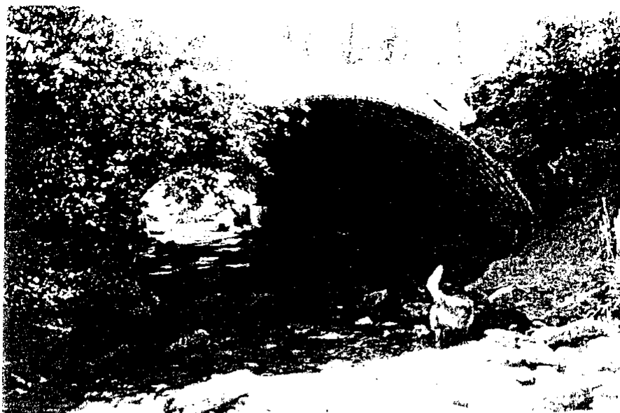
Photograph 9. Pipe arch culvert in Section 6 of Hospital Creek.
