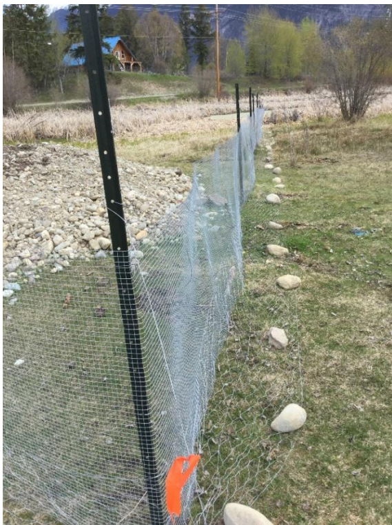
Figure 5. Horizontal fence woven into upright fencing to prevent predators from digging under vertical fence.
