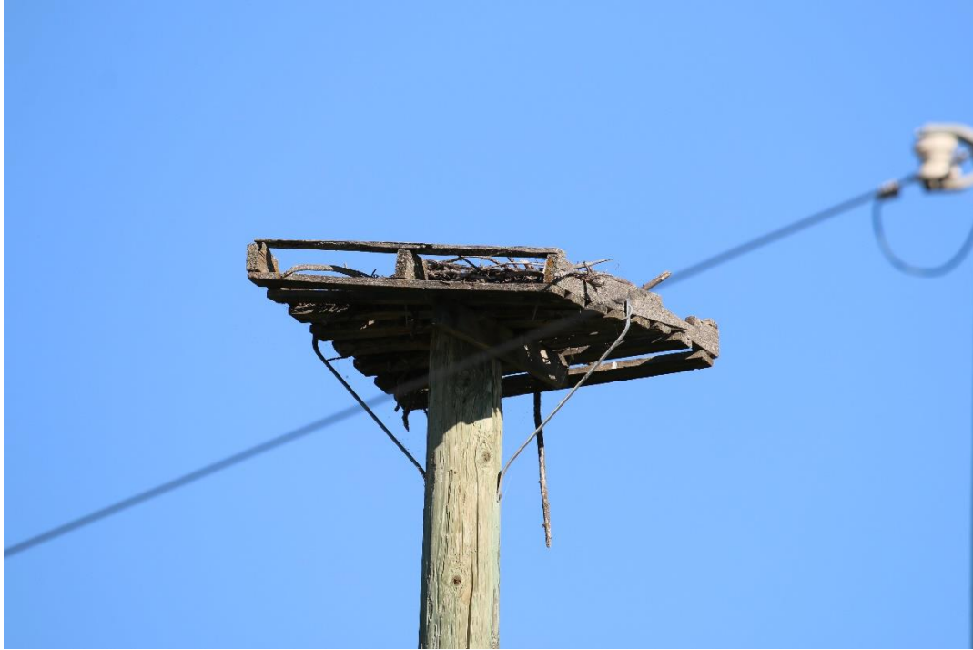
Figure 18. Deteriorating nest platform on a nesting pole in Radium.
