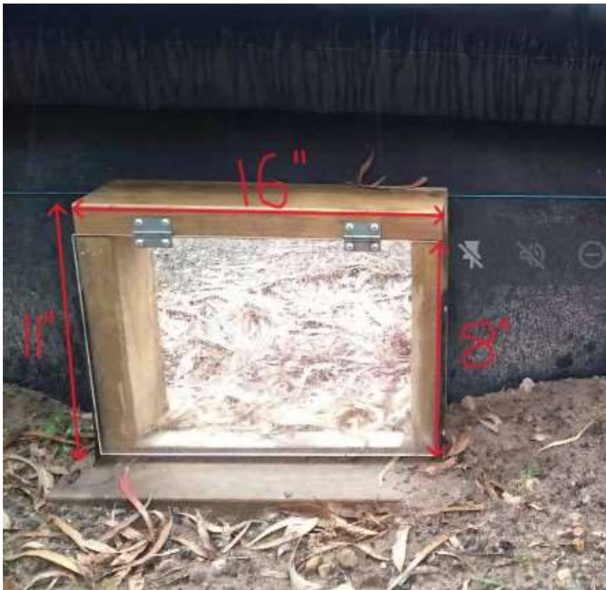
Figure 3. Dimensions and design for one-way escape doors.
