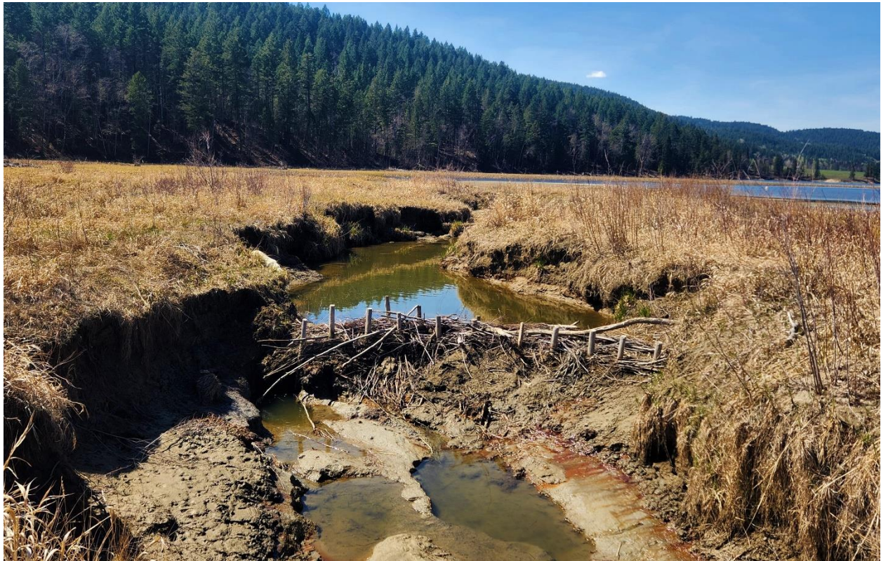
Figure 5: Beaver dam analogue built by CWSP in Site 38 in fall 2021. Photograph from early May 2023.
