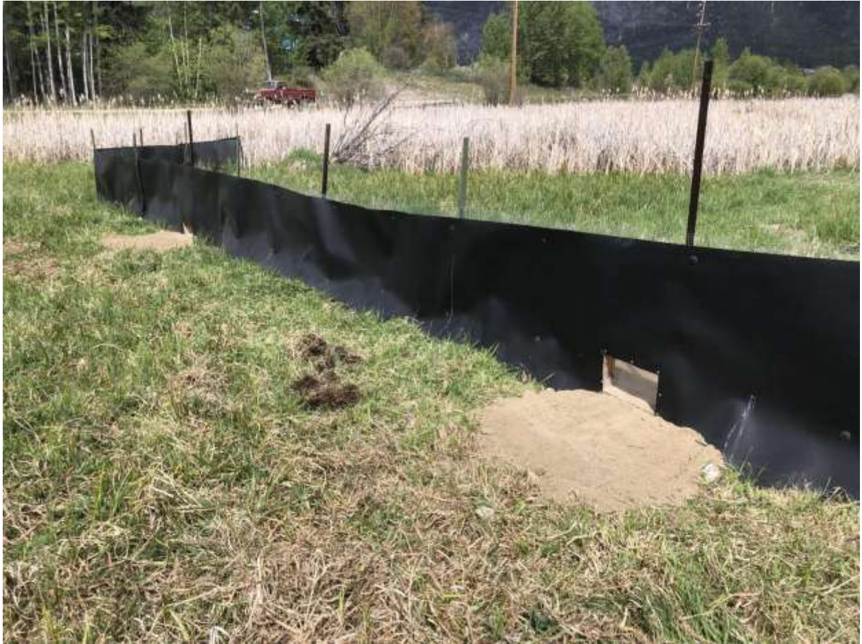
Figure 11. Improved ramps with landscape fabric under substrate to prevent weed growth at one-way escape doors.
