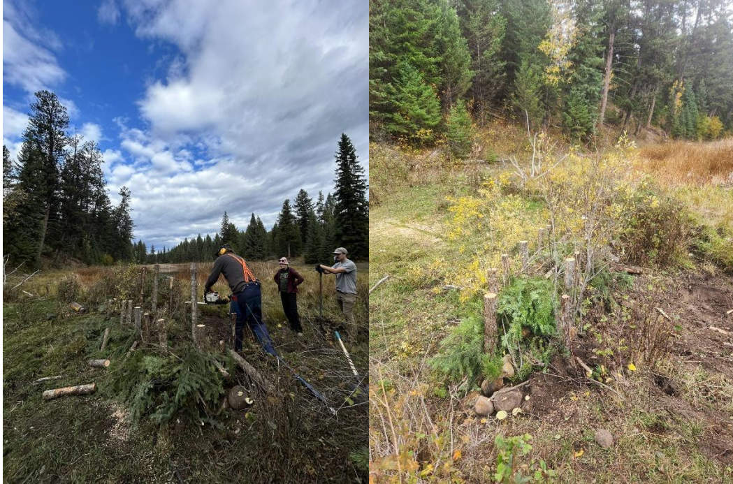
Figure 16. Cutting posts to appropriate height (left) and completed dam (right) at lower Beaver Channels dam (Location 1). Oct 8, 2024.
