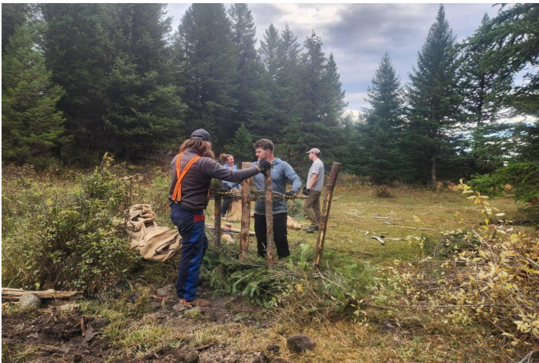
Figure 13. Weaving vegetation between posts at Beaver Channels' upper dam (Location 2).
