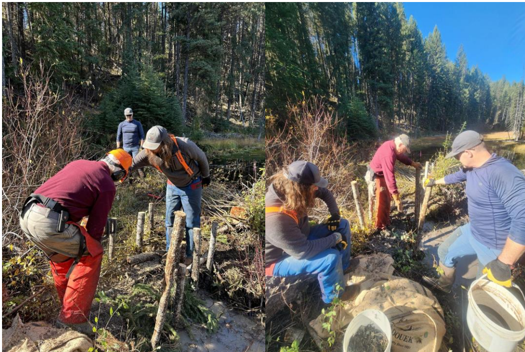
Figure 8. Lower S-land dam (Location 2) during construction, cutting down the posts to required height (left) and infilling the dam with mud and vegetation (right). Oct 7, 2024.
