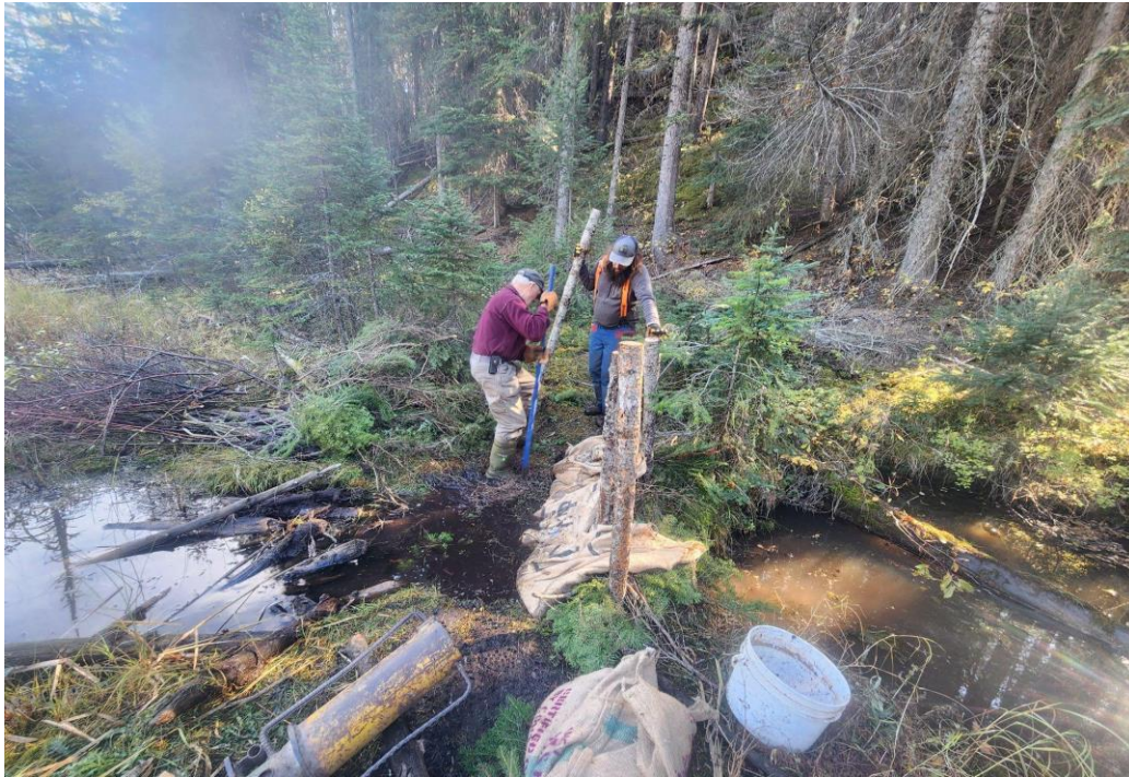
Figure 5. Pounding posts into the ground at S-Land upper dam site (location 1) during the construction.
